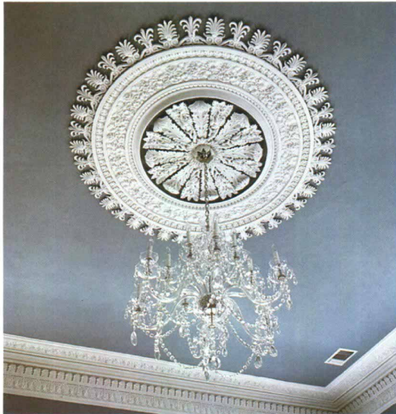
The author designed this new 6-ft. medallion for the parlor of a 19th-century Charleston house by analyzing the design of the house's original medallions. Ornaments from the cornice reappear in the outer circular band of the medallion; the center cluster matches those found in the extant medallions.
