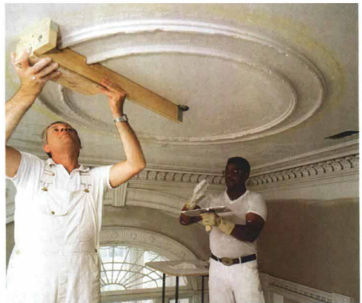
Assistant Richard Taylor trowels on a mixture of lime putty and plaster ahead of the template. It takes many passes with the template and some stuffing—swabbing plaster on rubber-gloved fingers—to eliminate voids.
